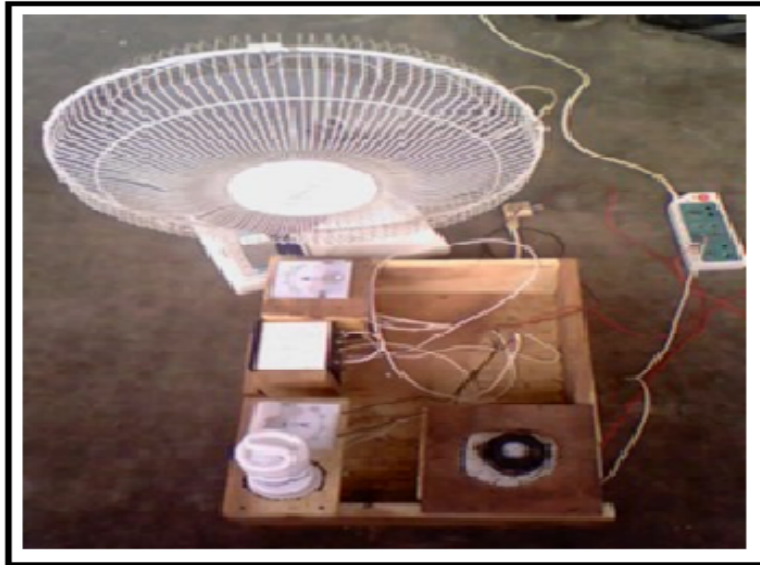
Figure 10: Measurement of power factor with inductive load
